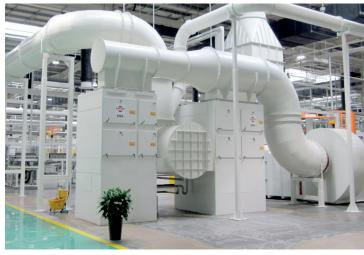
Dust extraction of a truck-engine production with a volume flow of 140 000  $\mbox{m}^{3}/\mbox{h}$
