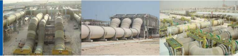
All FPI products are manufactured in accordance with stringent customer specifications and the most demanding international standards, using the latest technology, FPI offers the largest and most versatile large diameter fiberglass pipe product range in the market today. With diameters ranging from 12mm up to 4000mm, with an ability to withstand immense pressures of up to 3000 PSI, FPI's fiberglass-composite non corrosive pipe systems can transport water, oil, gas and petrochemicals including
